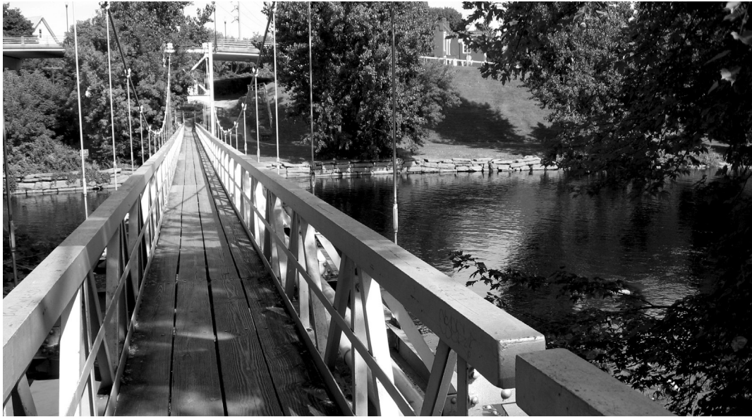
Saranac River Pedestrian Bridge. Photograph by Robin Brown
