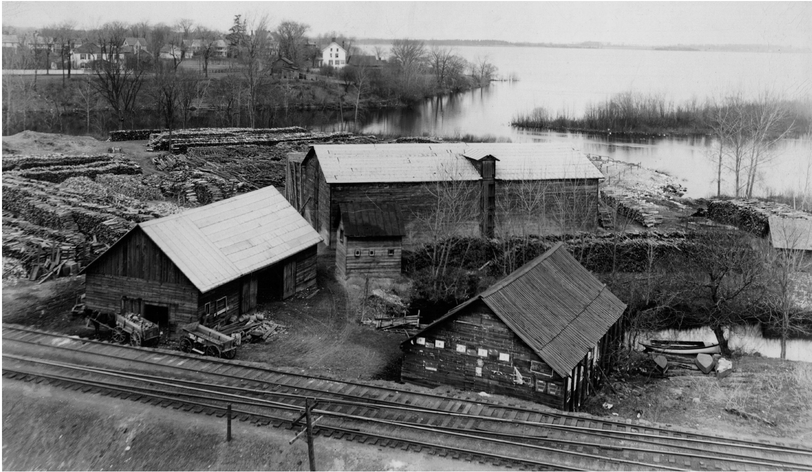
Lumber mill at mouth of Saranac River. (Clinton County Historical Association)
