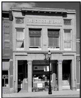
105 S. Main Avenue Citizens Bank Building, N&SHR
