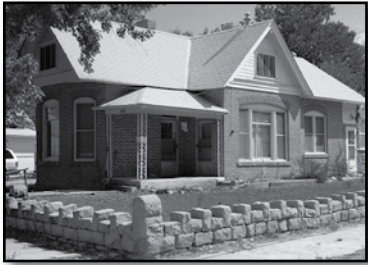
120 S. Church Avenue Vaughan-Eubanks House
