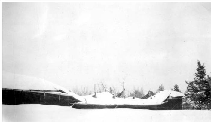
The roof of the Crystal Pool collapsed under the weight of two metres of snow in December, 1929.
