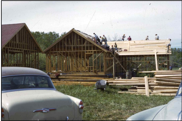
Work on the new camp went quickly with volunteers and professional contractors working side by side. (Photo: Raymond Historical Society)
