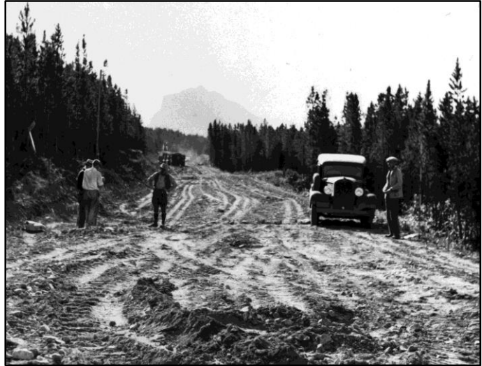
In places the progress toward the international border was easy to gauge by Chief Mountain which dominates the skyline. (Photo: Parks Canada)
