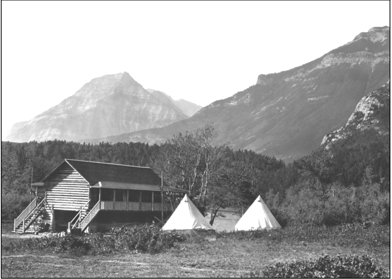
The first bath house, built for swimmers at Linnet Lake, was sited partially on what was once known as Moccasin Flats. (Photo: WLNP Archives)
