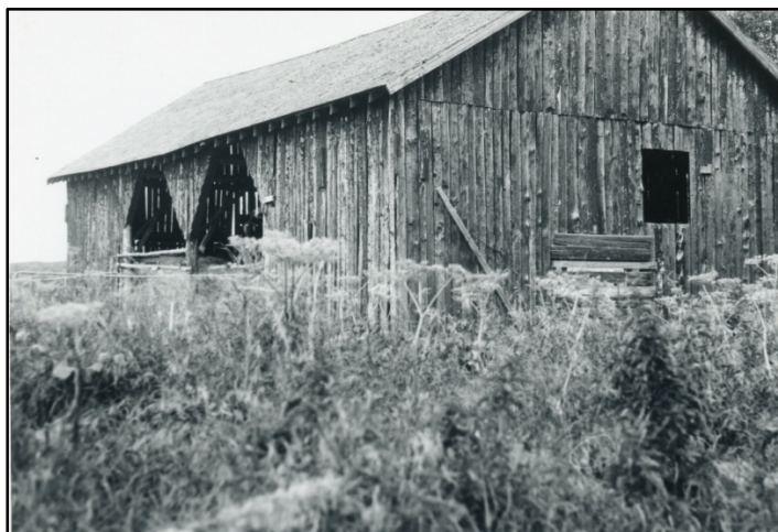
The Hay Barn, once located on the Blakiston Fan at the end of its namesake road, provided storage for the harvest. (Photo: WLNP Archives)
