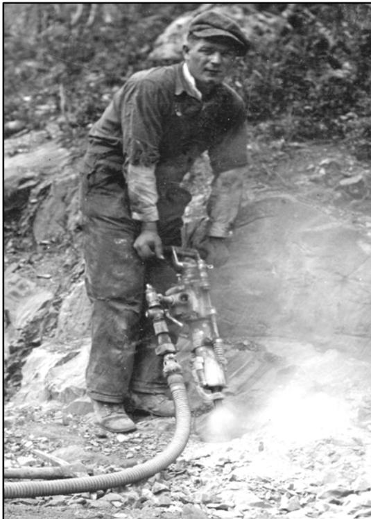
*Without benefit of any safety equipment, a workman uses a jack hammer to assist the 1920s construction of the Akamina Parkway. (Photo: Harwood Collection, WLNPA Archives)*
