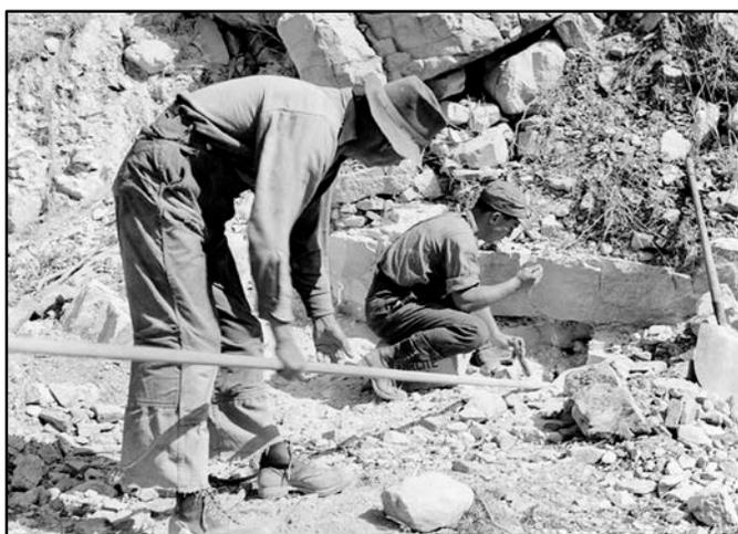
*Packing dynamite into the cliff face during 1948 blasting operations on the Akamina roadway.
