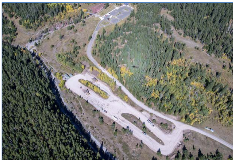
The redevelopment of the lower parking lot at the end of the Red Rock Parkway was completed in autumn, 2015 to provide more parking at this popular visitor destination. (Photo: Parks Canada)
