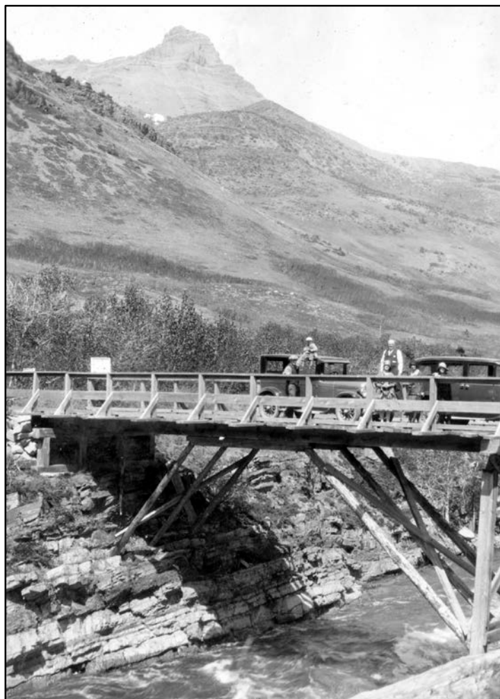
Upper Pass Creek Bridge allowed access to the Crandell Lake trailhead. The structure has been replaced many times, the latest being in 2015.
