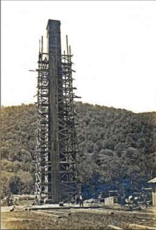
Acid Factory Chimney construction 1912
