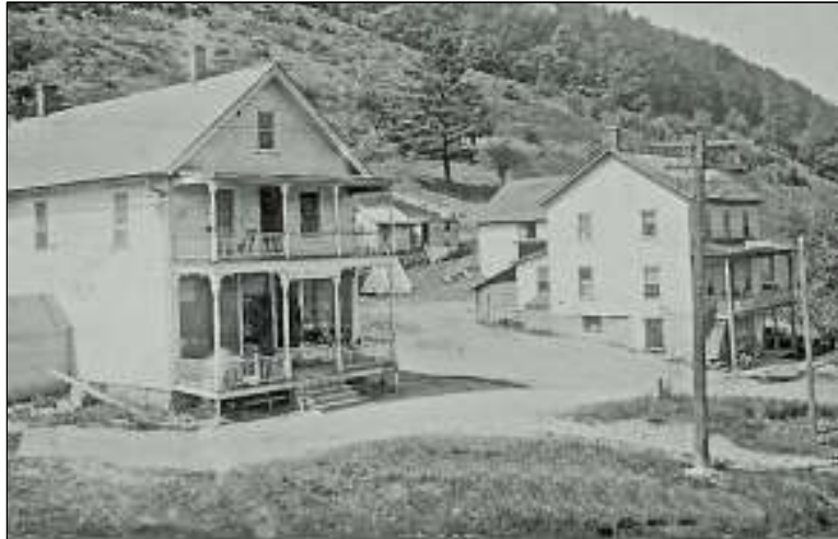
Hotel Leroy –Johnson Store and Post Office 1914
