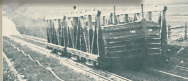
An empty cradle car sits in the water at the bottom of the inclined plane.
