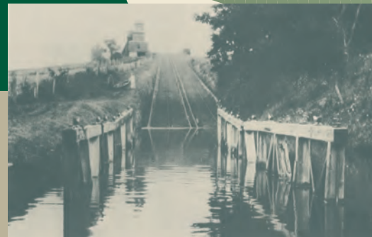
An empty cradle car sits in the water at the bottom of the inclined plane.
