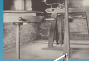
A historic view of the controls used to operate the inclined plane.
