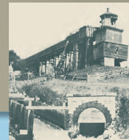
The Plane 9 West power house is seen above, while below water flows from the bypass trough on the left and the tailrace tunnel on the right.
