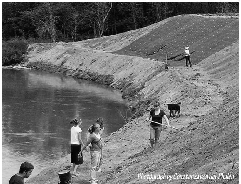
Volunteers begin laying erosion mat on the river bank.
